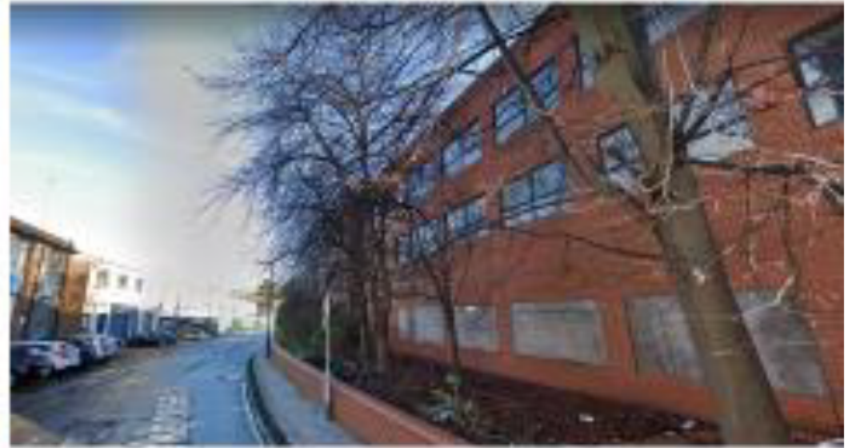
Existing building 10-12 Parkhouse Street
