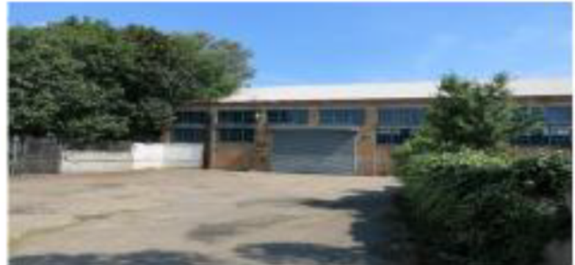
Existing yard rear of 1-13 Parkhouse St
